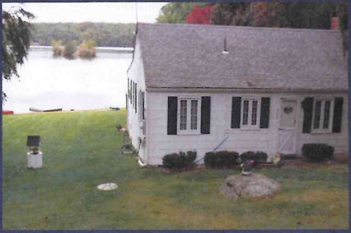
Typical Grinder Pump Location
